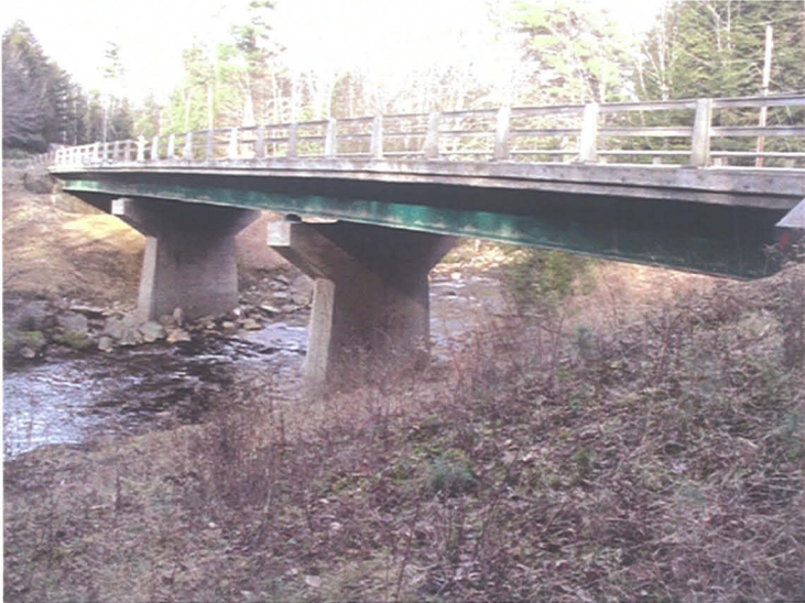
Downstream Elevation of Bridge at Low Water
